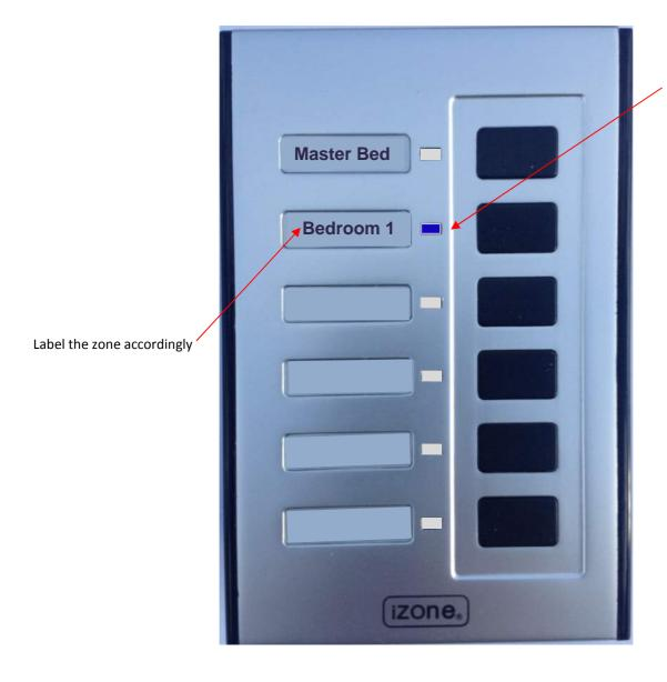
Switch all zones OFF and one zone ON. Check which zone is being supplied with air.
